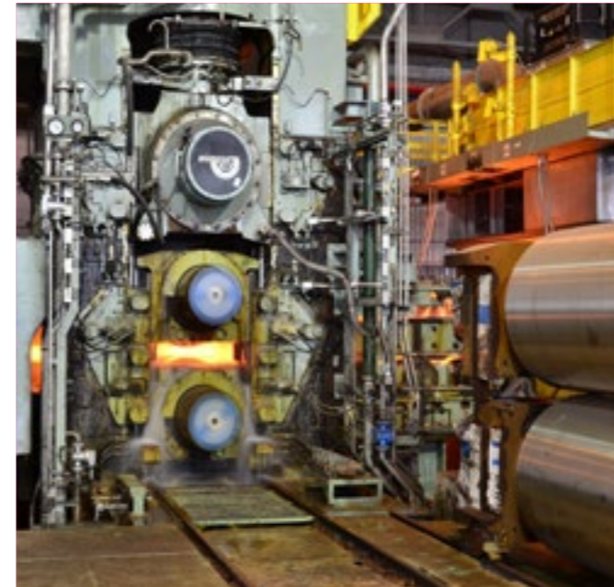
Roughing mill at USIMINAS, Cubatao No.2 HSM, Brazil
