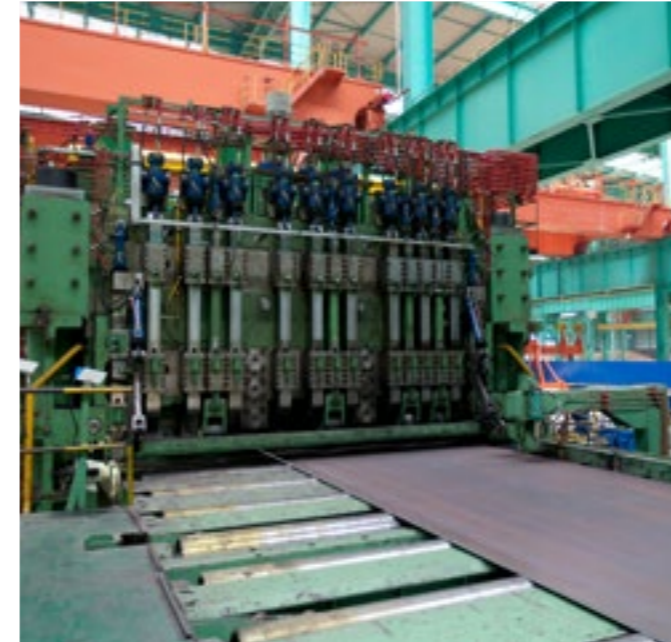
Divide shear at Dongkuk Steel, Dangjin, South Korea
